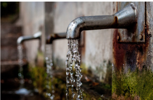
Domestic Water Supply
